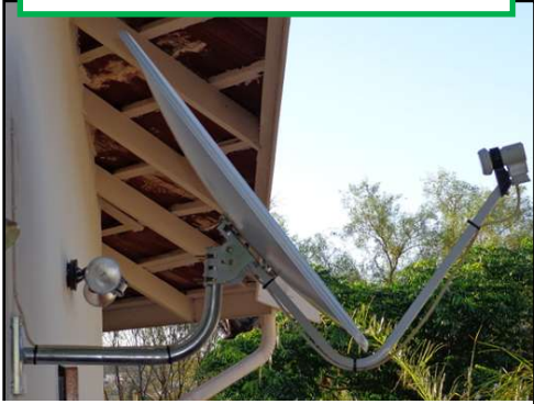
Figure 7 - Incorrect and correct offset dish elevation (applicable for Namibia and South Africa)
